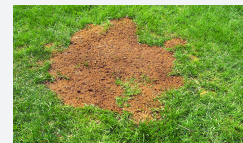
Temporary backfilled holes in your yard are filled with soil and left to settle.
